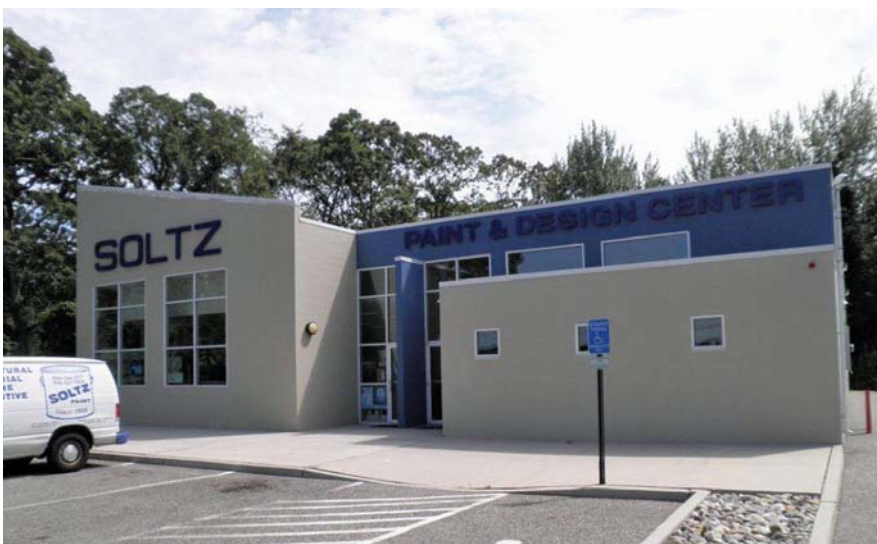
● The Cape May Court House store was built from scratch and features contemporary architecture and a striking exterior paint scheme.
